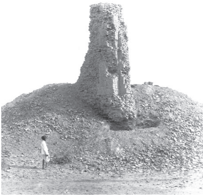
▲ Figure 3. Henry Cousens' 1897 photo (Cousens 1929) of the ruined tower at Brahmanabad (Bhamanabad), whose excavation had been first reported by Bellasis (1857a, b; Cousens 1905). Crushed skeletons and scattered coins indicate its destruction by an earthquake within the decade or so following A.D. 975, the date of the youngest coins buried at the site.
